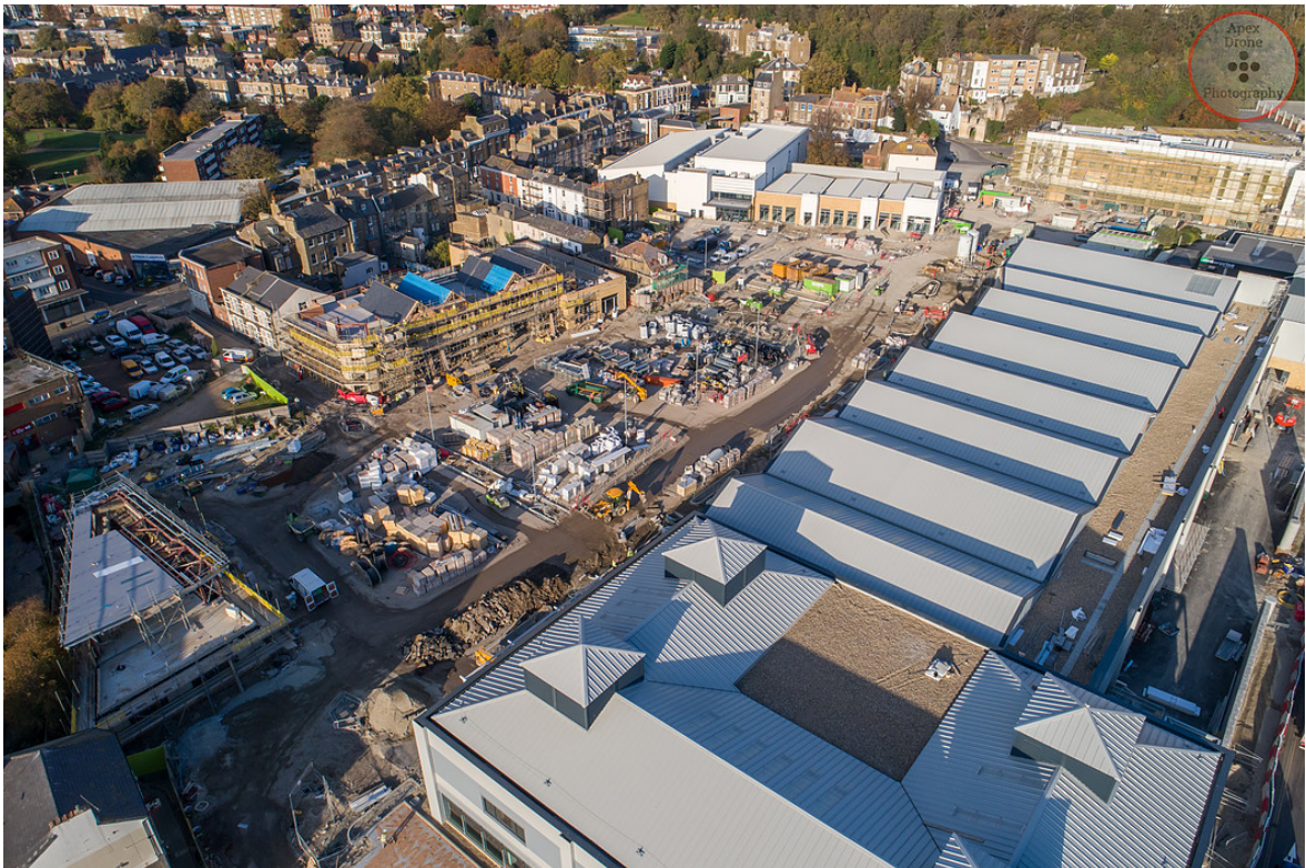
Figure 11.4 Aerial view of the St James's site in progress (Photo courtesy of Apex Drone Photography)
